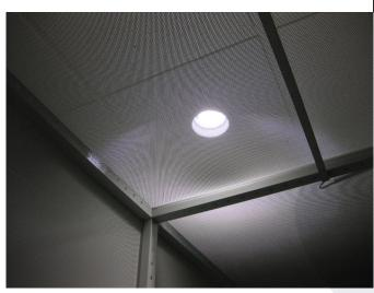
Perforated panels also allows for light (and air) from the outside environment to pass through the shielding, giving the patient the view of a bigger room. A dedicated HVAC system is not needed.
